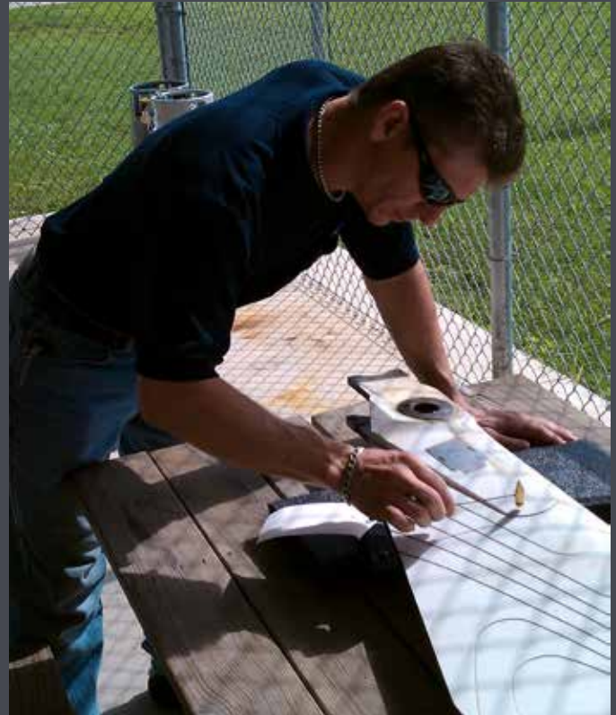
CTI technician performing on-site repairs
